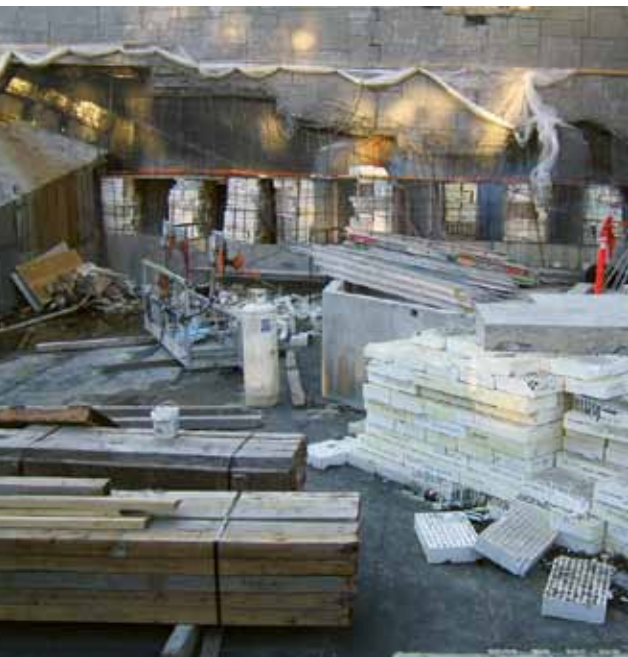
THE OBELISK TOWER, COQUITLAM, B.C. – LANDSCAPING CONSTRUCTION BY TERRA DESIGN INC.
