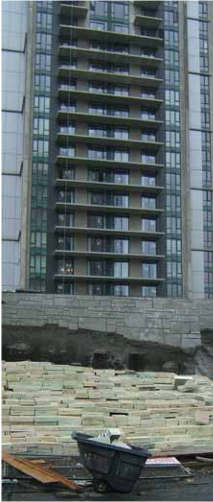
Figure 4. Terracotta has been placed to create a stepped slope. Note the mix of tray sizes and the rough construction. Trays can be broken or cut with a handsaw to fill gaps.
