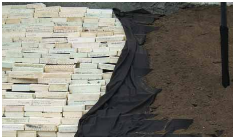
Figure 2. Nonwoven, nonbiodegradable landscape fabric can be used as the filter fabric above the drainage layer.
