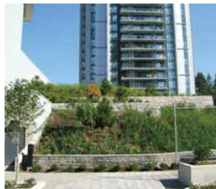
Figure 6. For a roof located in the city of Coquitlam, British Columbia, planting is initiated (A) and completed (B). The completed site in mid-August 2008, less than a year later (C). Note that only a single mortality has resulted.
