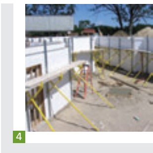
4 Brace the wall
